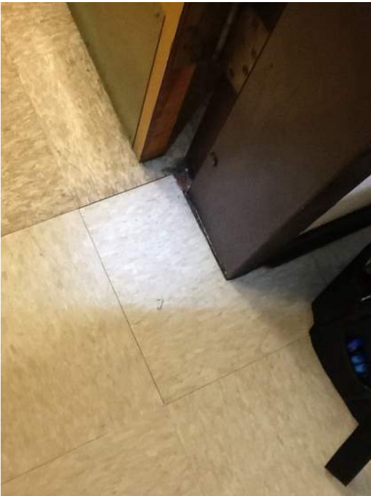
Photo 11: View of Homogenous Area 11 Room 111
