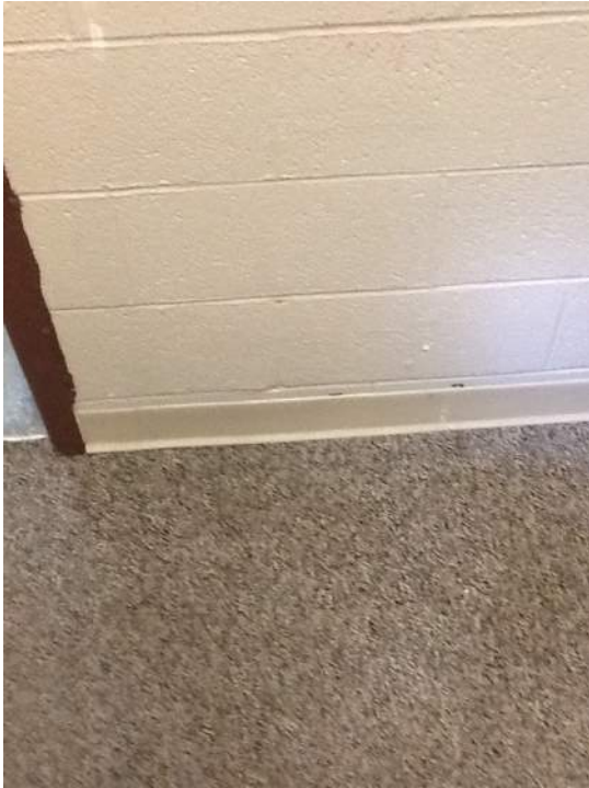
Photo 9: View of Homogenous Area 9 Room 108
