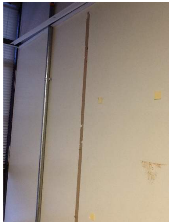
Photo 4: View of Homogenous Area 4 Room 103
