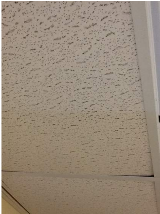
Photo 5: View of Homogenous Area 5 Room 103
