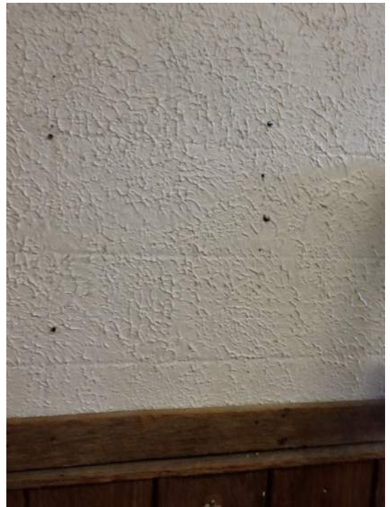
Photo 8: View of Homogenous Area 8 Room 105
