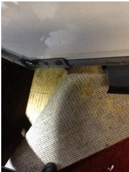
Photo 7: View of Homogenous Area 7 Room 105
