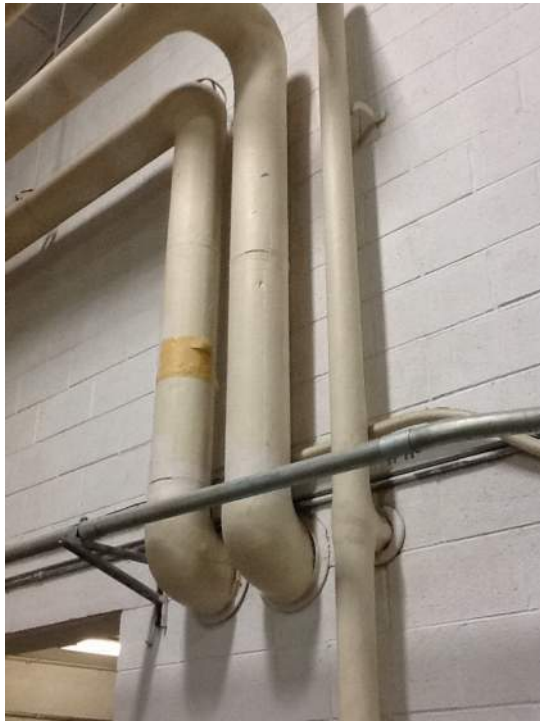
Photo 1: View of Homogenous Area 1 Room 101
