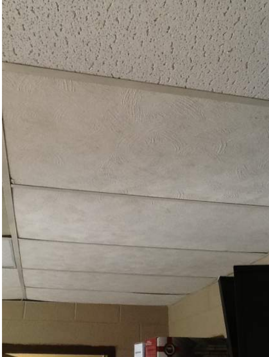
Photo 13: View of Homogenous Area 13 Room 120
