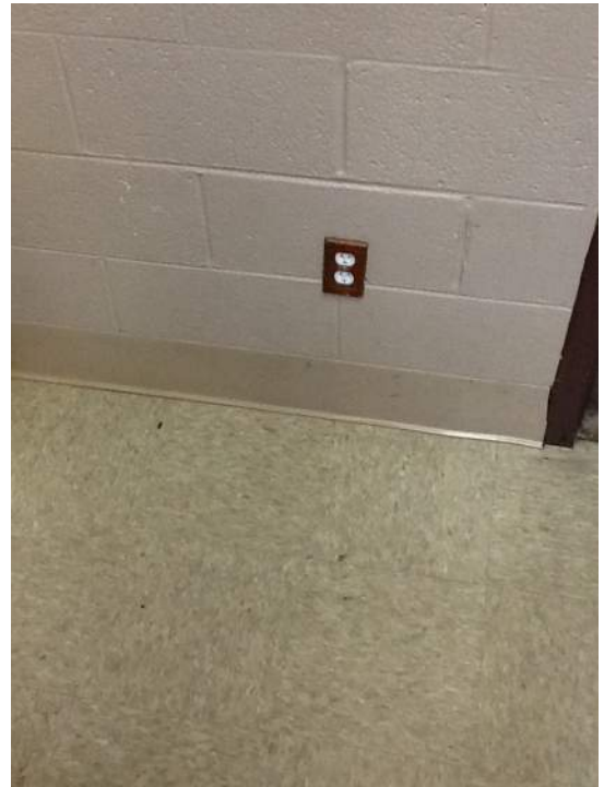
Photo 2: View of Homogenous Area 2 Room 102
