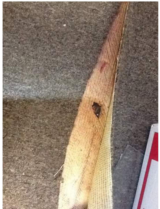
Photo 6: View of Homogenous Area 6 Room 103
