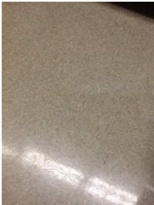
Photo 3: View of Homogenous Area 3 Room 102
