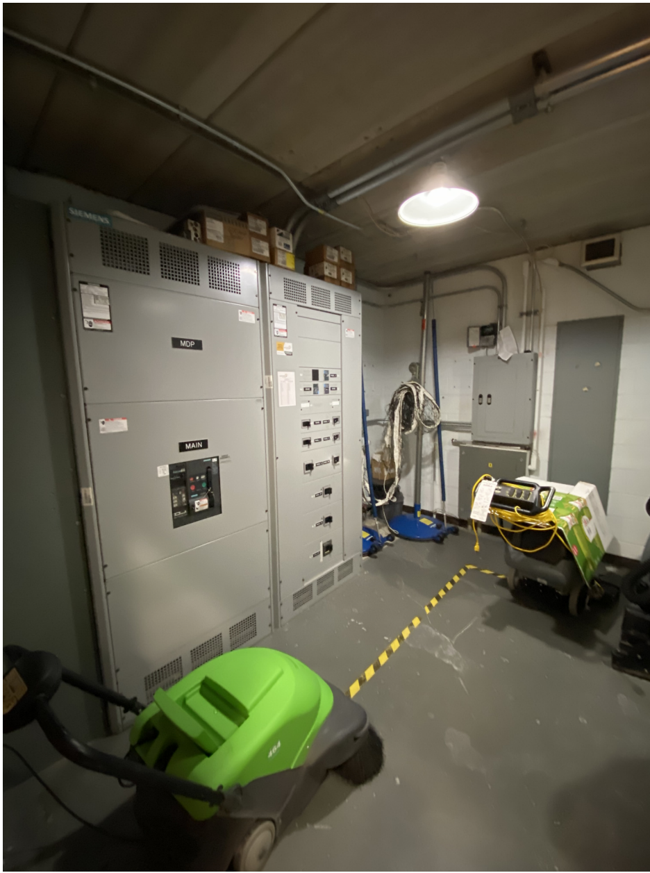
MDP LOCATED IN ELECTRICAL EQUIPMENT ROOM
