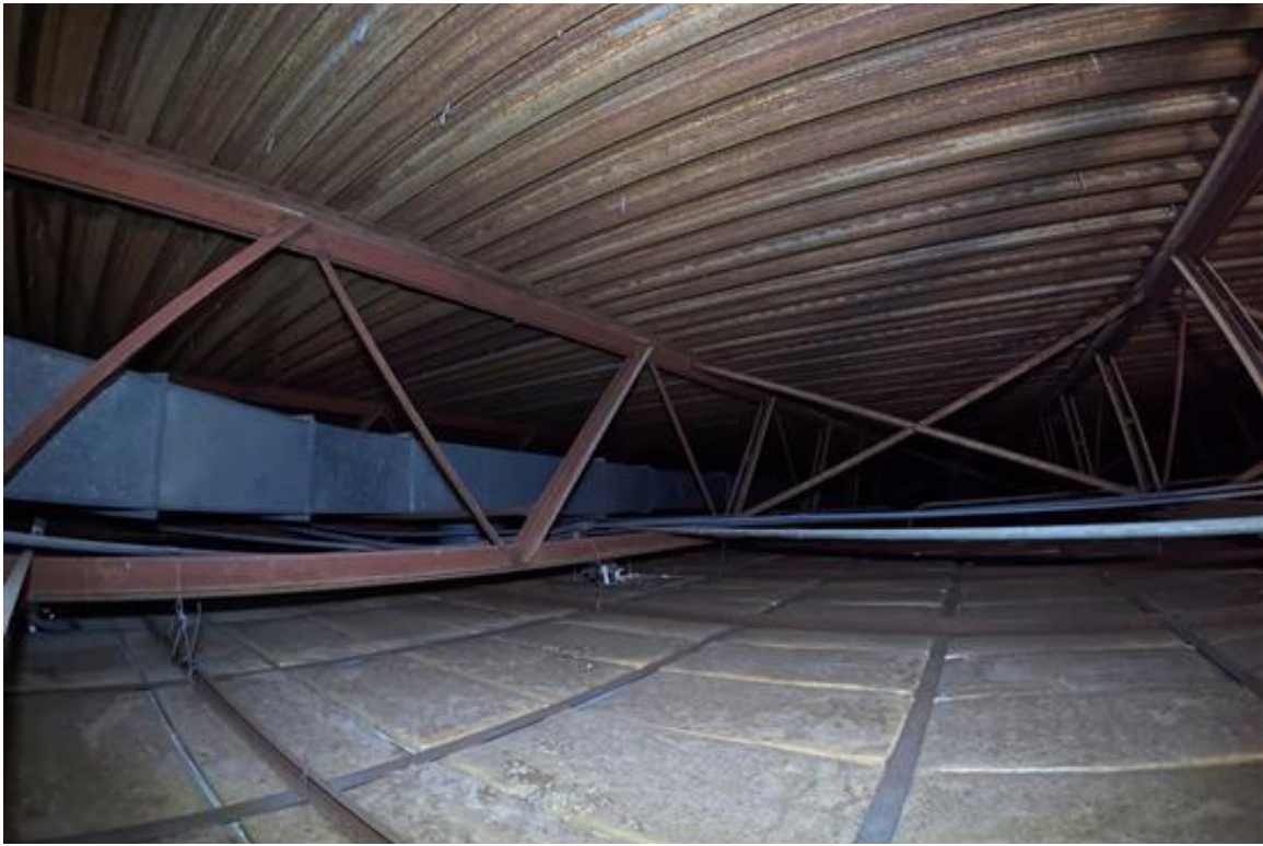
Photo 15 - The roof is framed with metal roof deck over long span steel roof joists.
