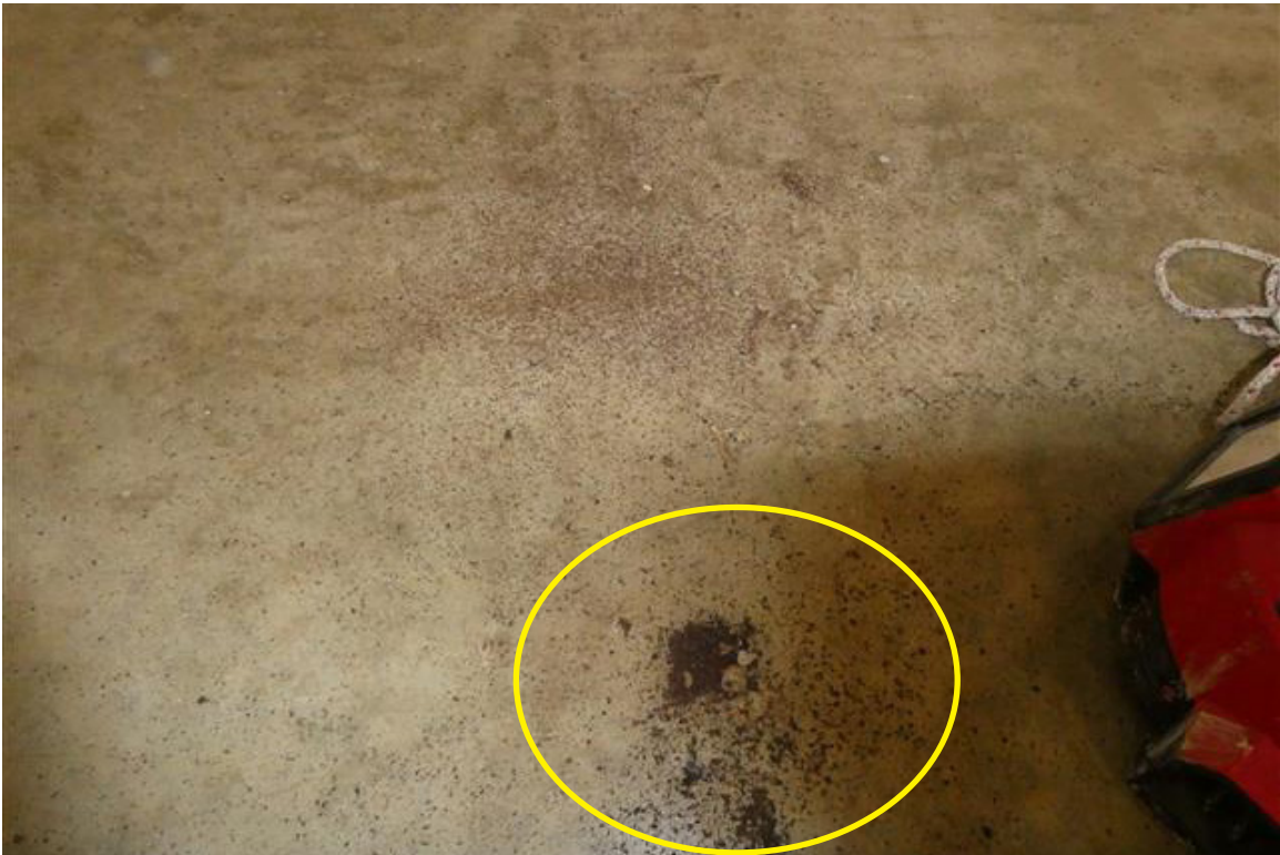
Photo 22 - Corrosion particulates fell from the ceiling as the tiles were removed.
