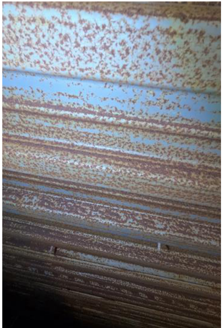
Photo 34 - We did not observe any locations where the deck had rusted through.
