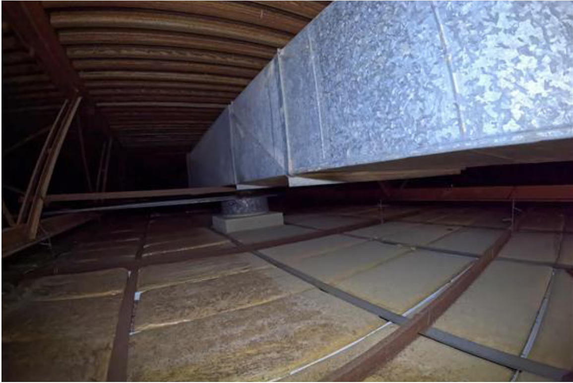
Photo 35 - The ductwork appeared to be in good condition.
