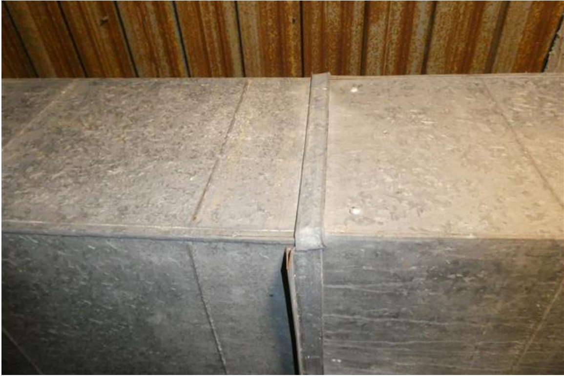
Photo 17 - The ductwork is constructed of galvanized metal.
