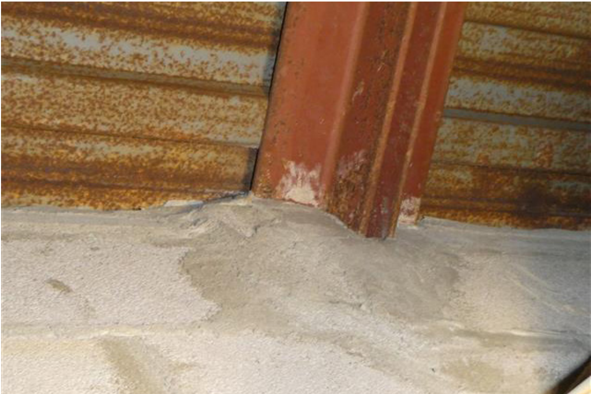
Photo 30 - The red primer remains on most of the joists.
