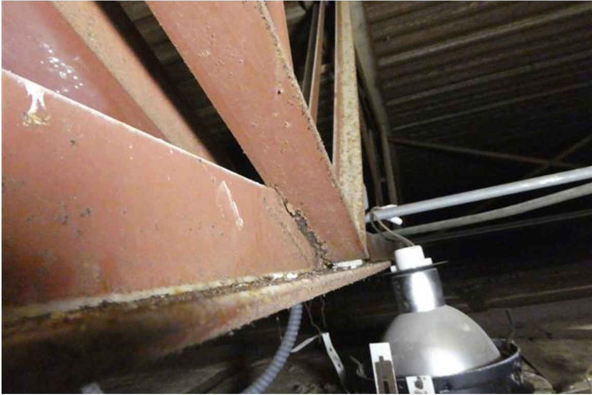
Photo 31 - Corrosion appears to be more advanced at welded connections in the joists.
