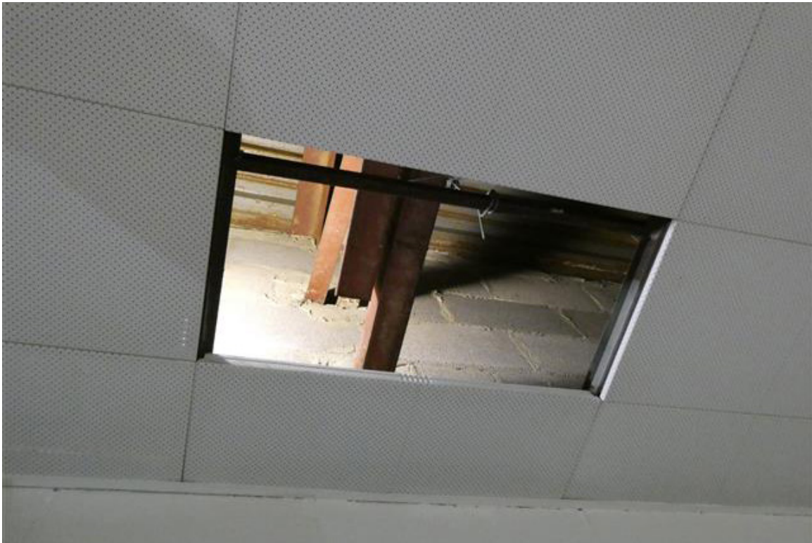
Photo 43 - The ceiling must be removed, either in whole or in part, to access the space above. Re-installing the ceiling tile was difficult given the expansive force on the entire ceiling and the corrosion product that has formed on the splines.
