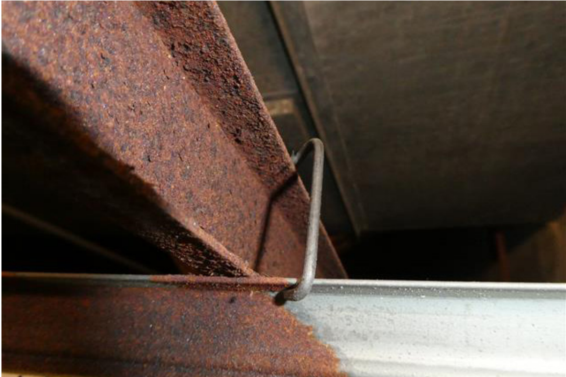
Photo 25 - The ceiling support structure clips...
