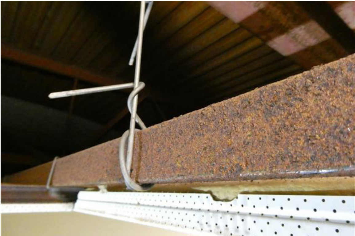
Photo 26 - ...and wires appeared to be in good condition and free of corrosion.
