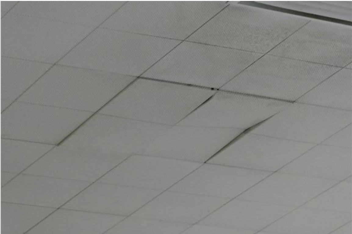
Photo 44 - One area, two tiles wide, appeared to have been removed and re-installed previously. These tiles were noticeable compared to the adjacent undisturbed tile.
