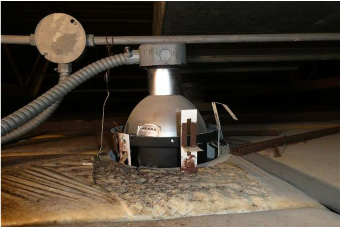
Photo 28 - ...and the lights themselves have corroded.
