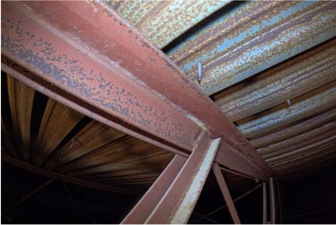
Photo 29 - Surface corrosion has formed on portions of the steel roof joists.
