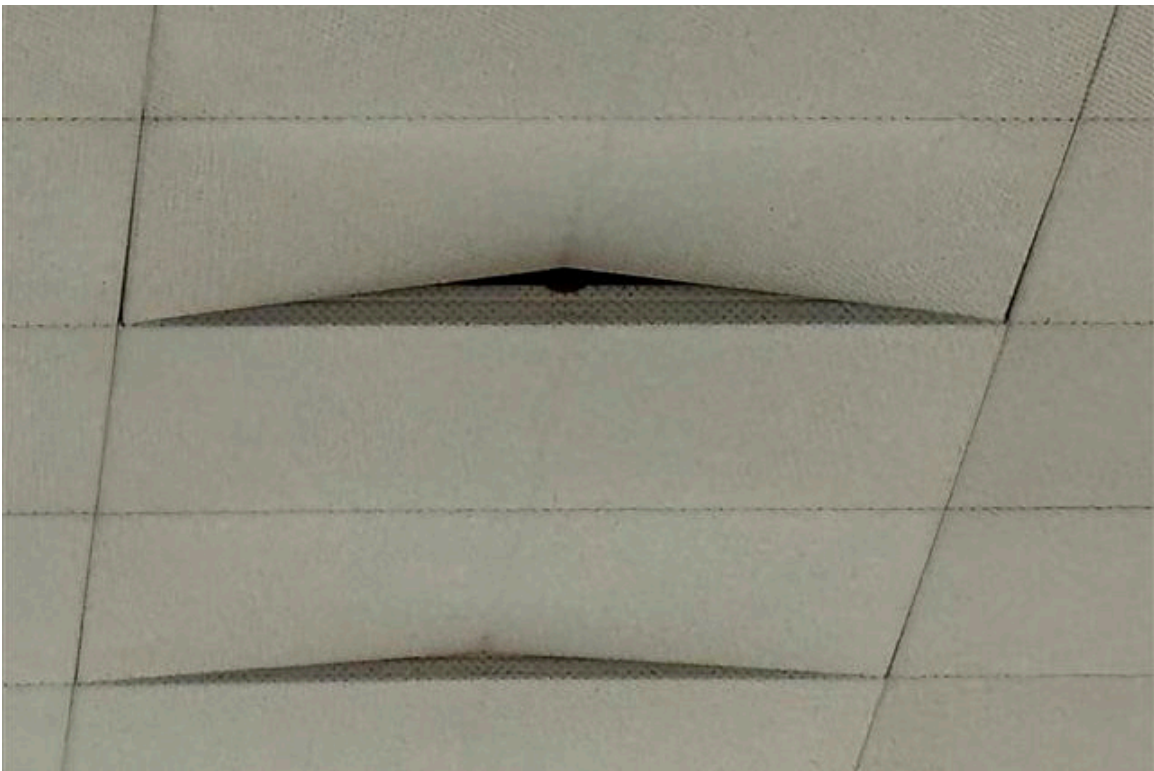
Photo 40 - As a result, numerous panels have buckled under the expansive forces from the warm pool area.
