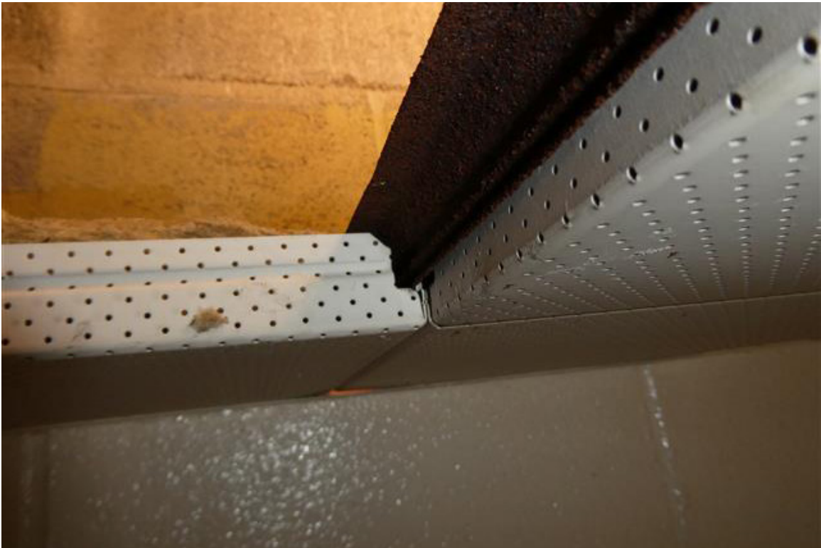
Photo 12 - These ends nest to the adjacent tile.
