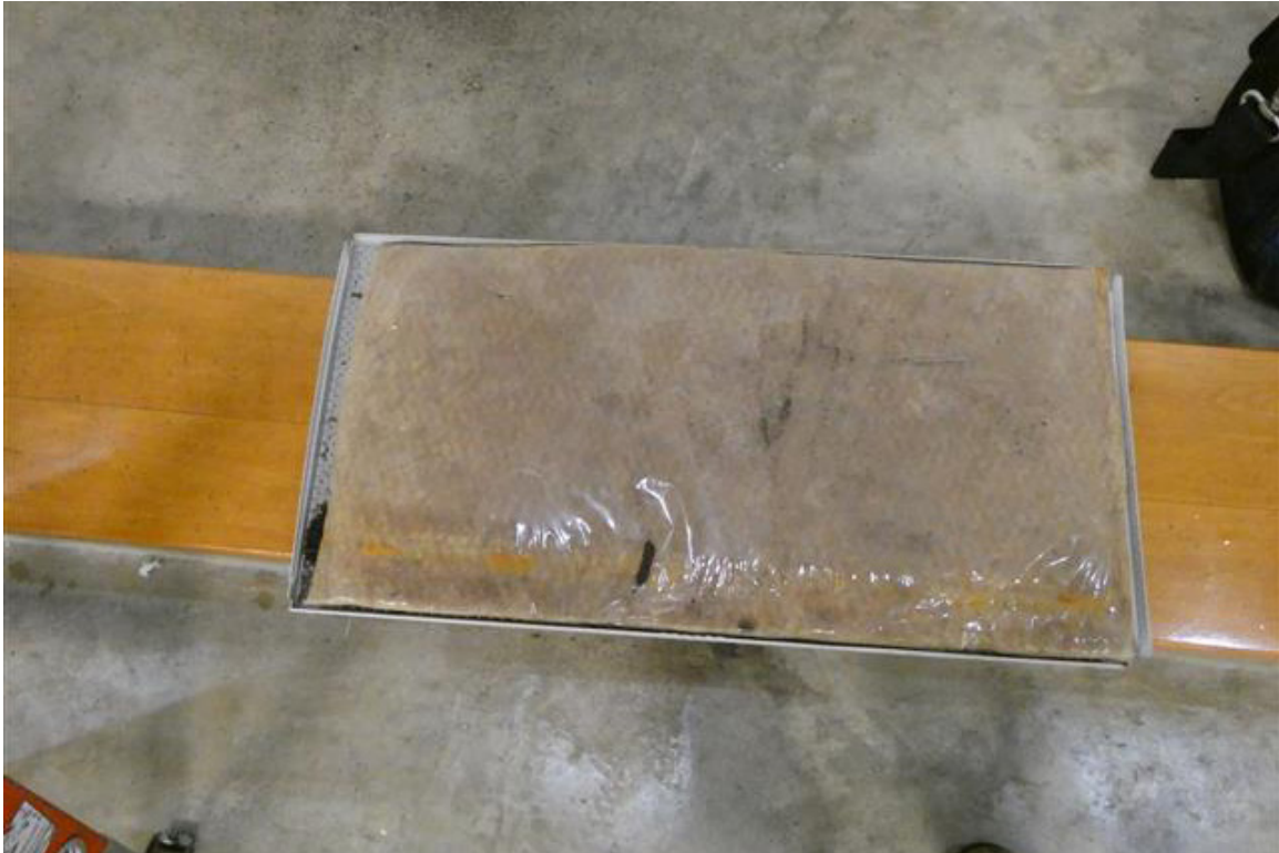
Photo 07 - The metal ceiling tiles are perforated and lined on the top side with insulation wrapped in plastic.
