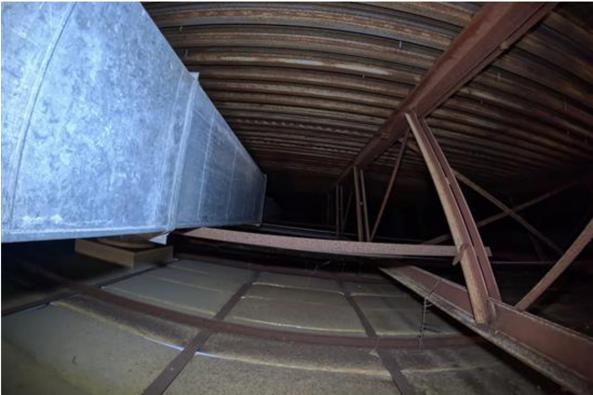
Photo 36 - The galvanizing remained, protecting the carbon steel as intended.
