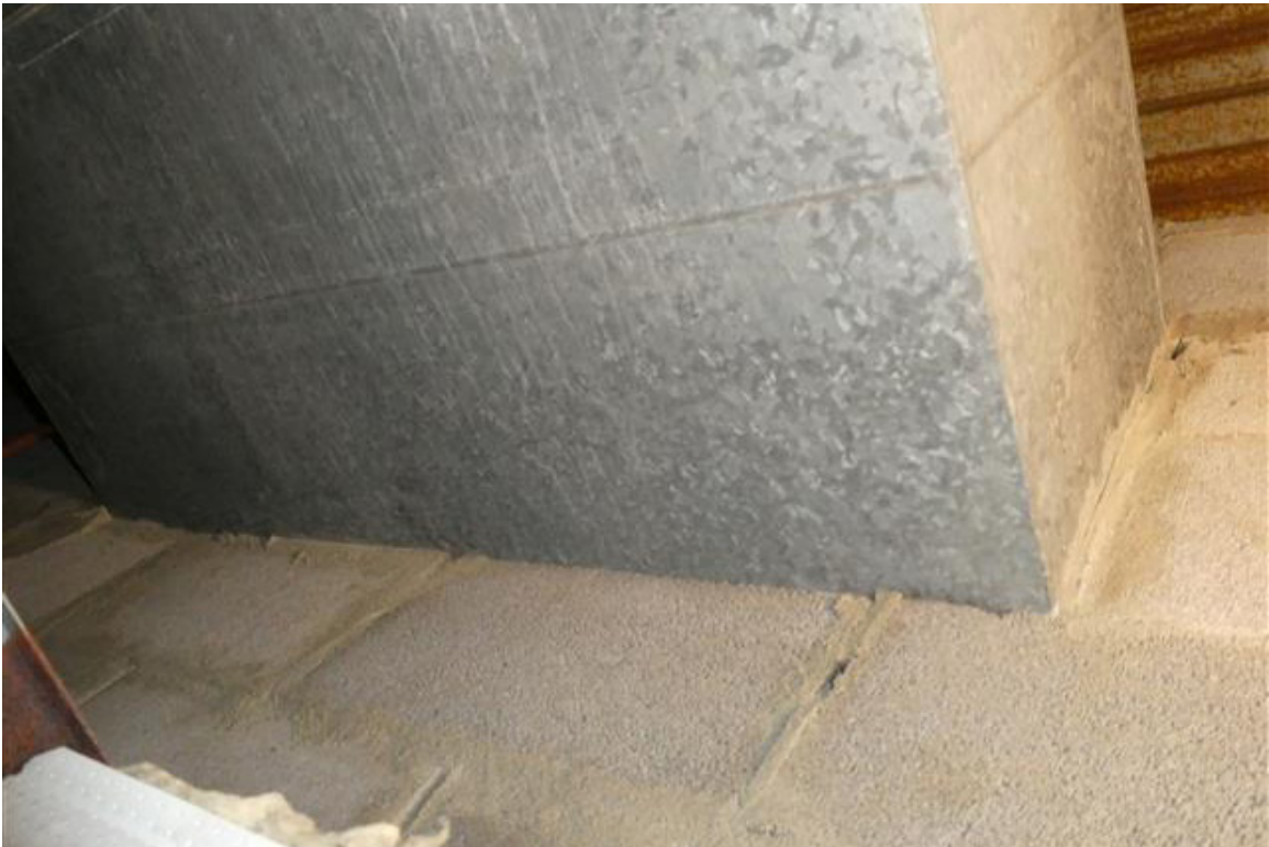
Photo 18 - The CMU of the plenum wall is cut to fit tight around the ductwork.
