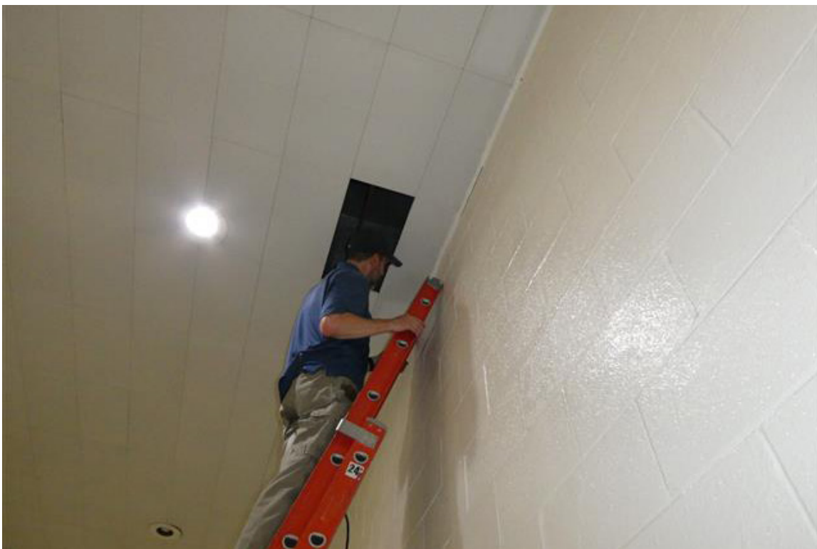
Photo 06 - A single ceiling tile was removed in three locations to view conditions within the interstitial space.
