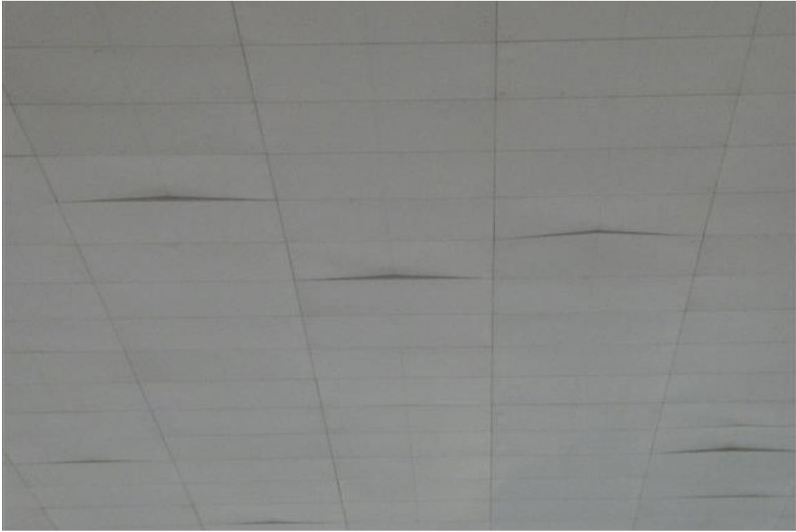
Photo 41 - The buckling occurs sporadically throughout the area.
