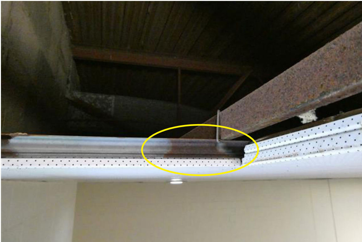
Photo 23 - Portions of the ceiling spline have corroded.
