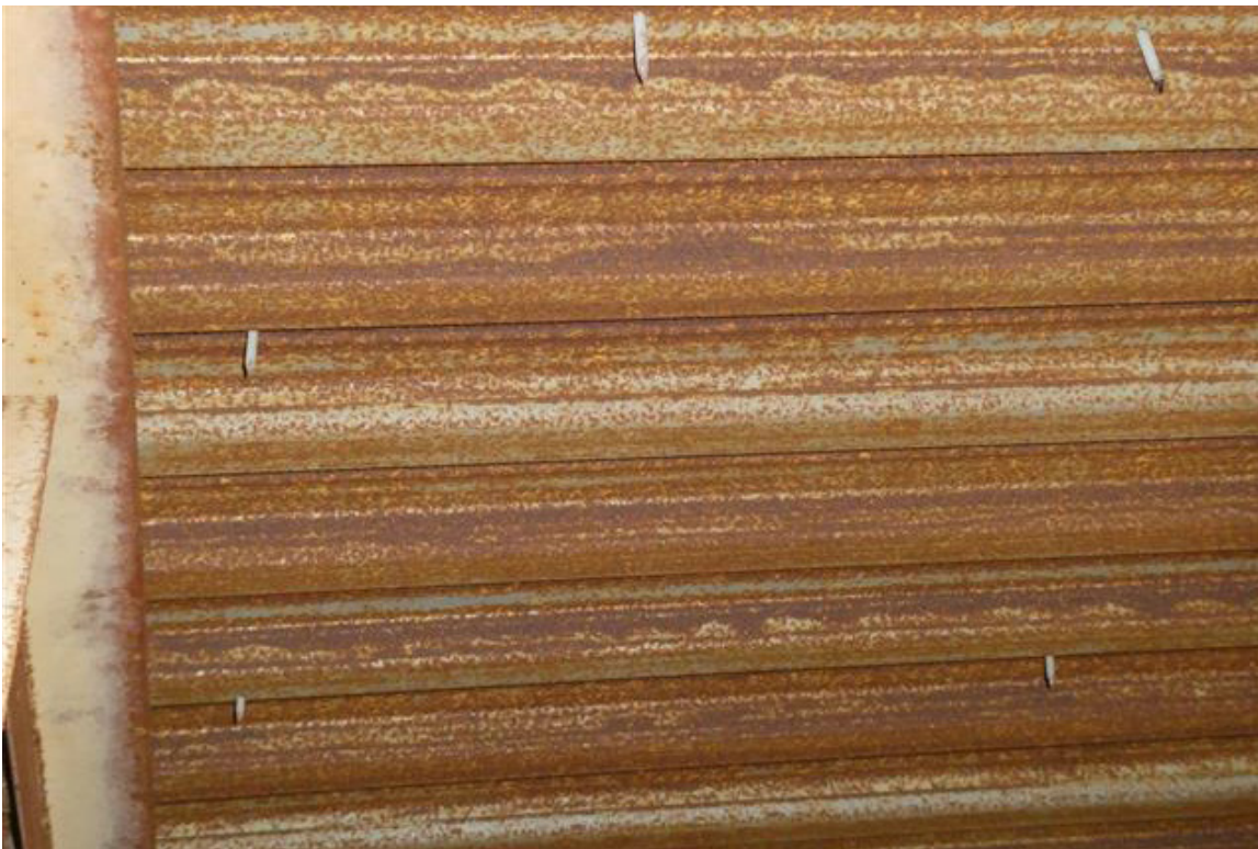
Photo 33 - Corrosion has formed on the underside of the metal roof deck.
