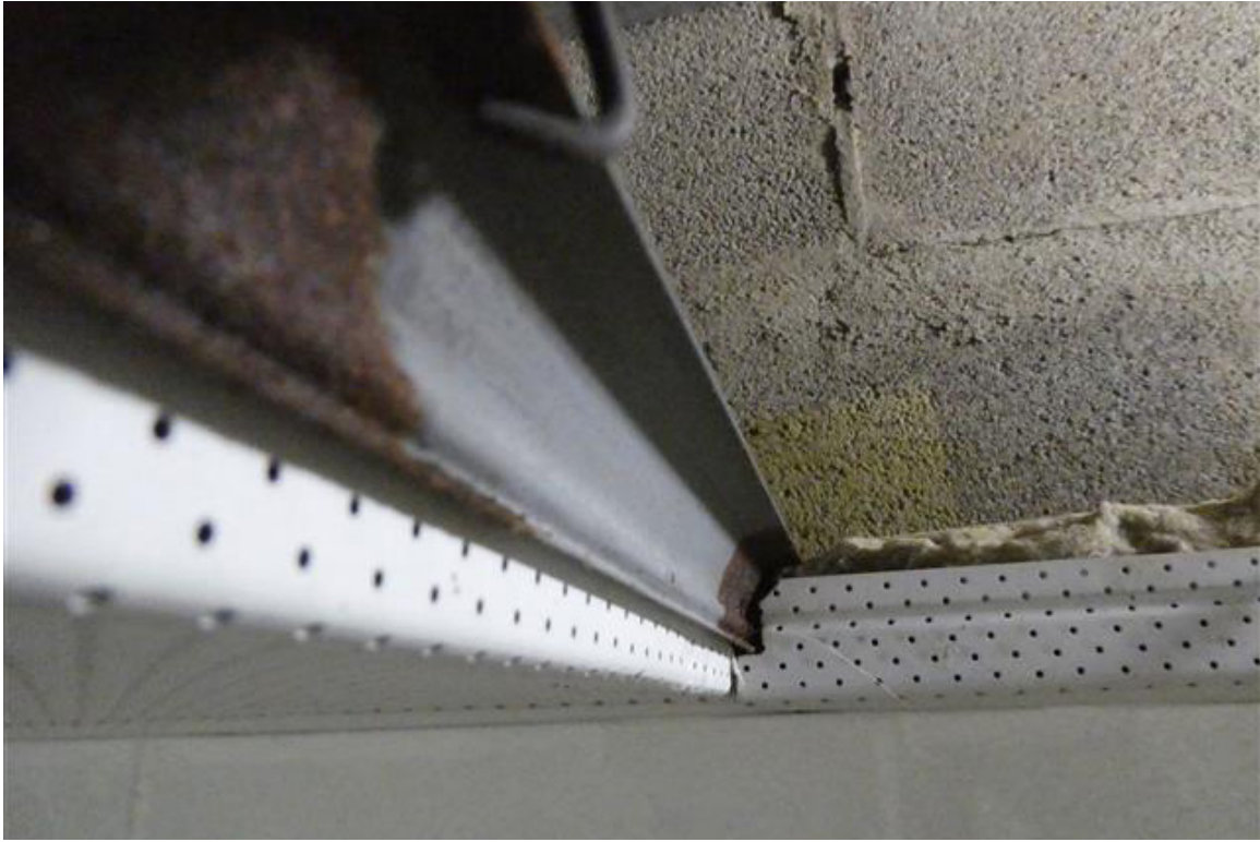
Photo 09 - The tiles are supported on the short edge by a concealed spline.
