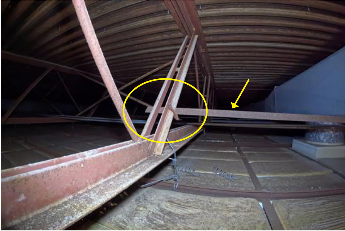
Photo 19 - The ductwork is supported by an angle member clipped to adjacent roof joists.
